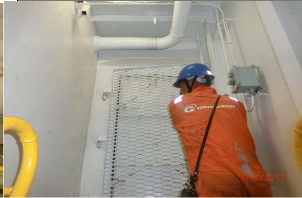
VERIFYING OTHER ACCESS ARE LOCKED
